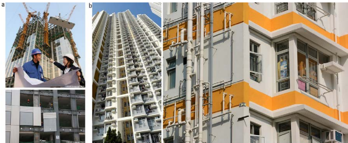
Fig. 2. (a) «J57 SkyTown». Photo: © BROAD Group via CTBUH [http://www.skyscrapercenter.com/building/j57-skytown/19743], (b) Public housing in Hong Kong. Photo: © Generalova Elena.
